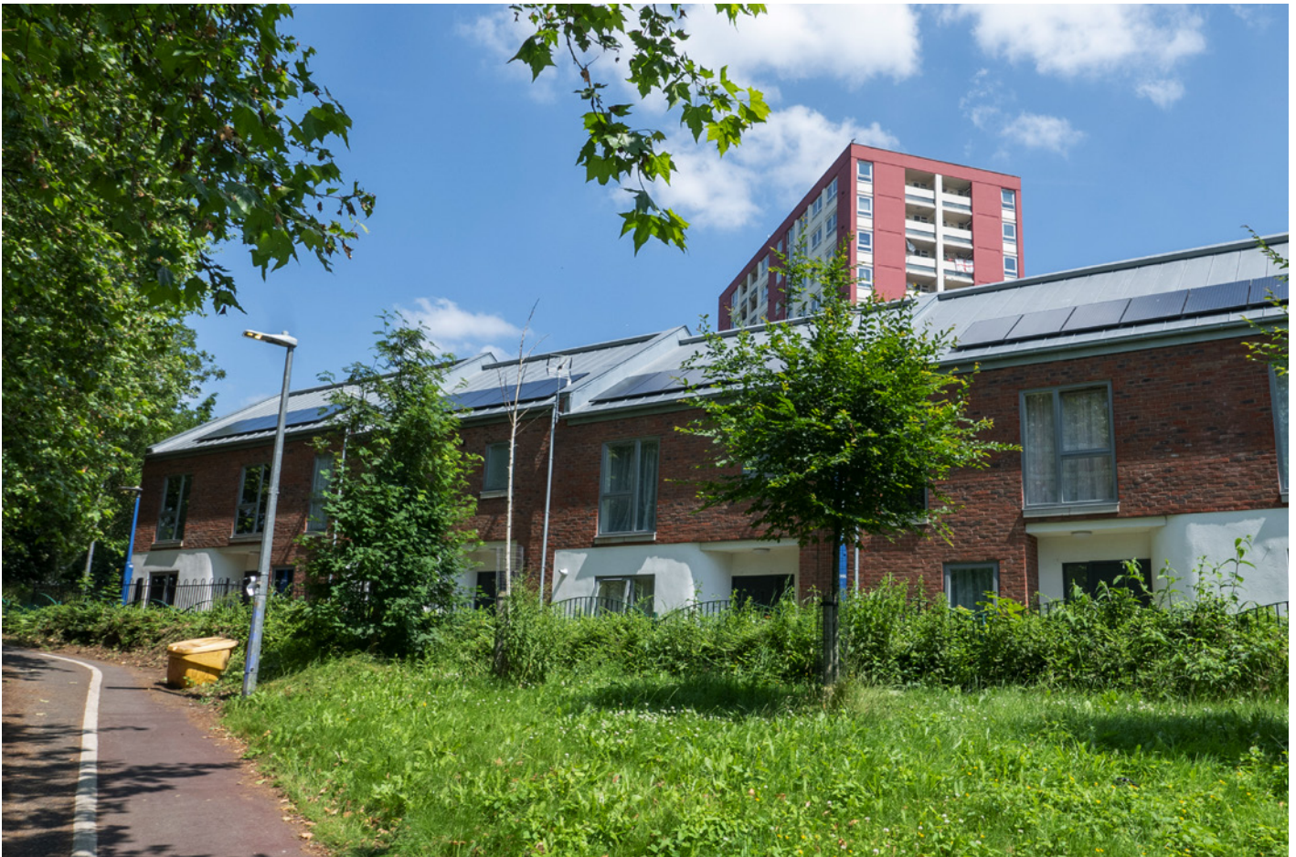
Solar panels on the roof of Barton Hill housing, Bristol © Bristol Design, Bristol City Council
