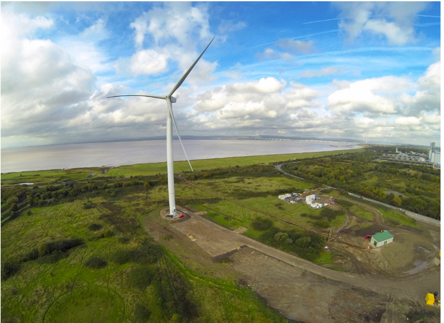
Bristol City Council wind turbine, Avonmouth © Bristol Design, Bristol City Council
