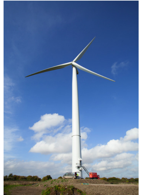
Bristol City Council wind turbine, Avonmouth © Bristol Design, Bristol City Council
